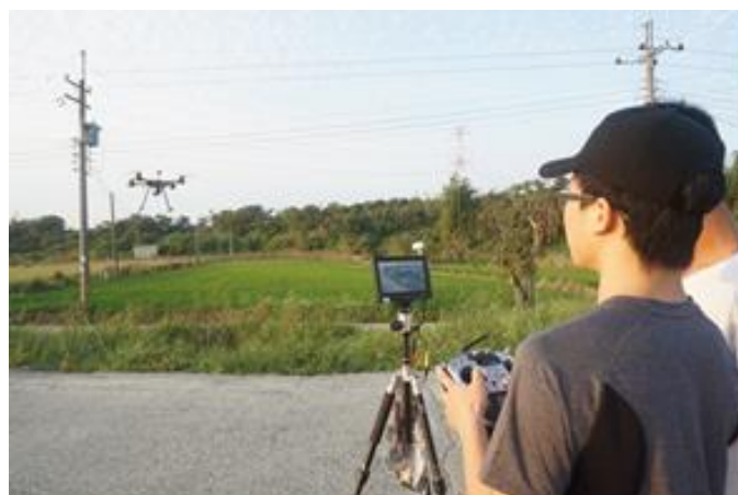
Fig. 2. UAS Power Line Inspection.
